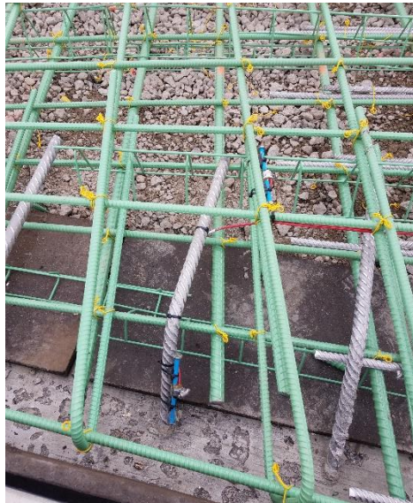
Figure 5.43. Story - Approach Slab Modified Subbase Condition Immediately before Concrete Pouring
