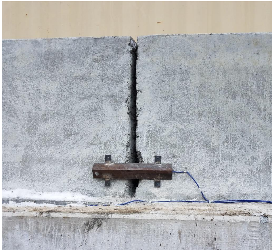
Figure 5.27. Story - Crackmeter Installation across the Barrier Rail Joint
