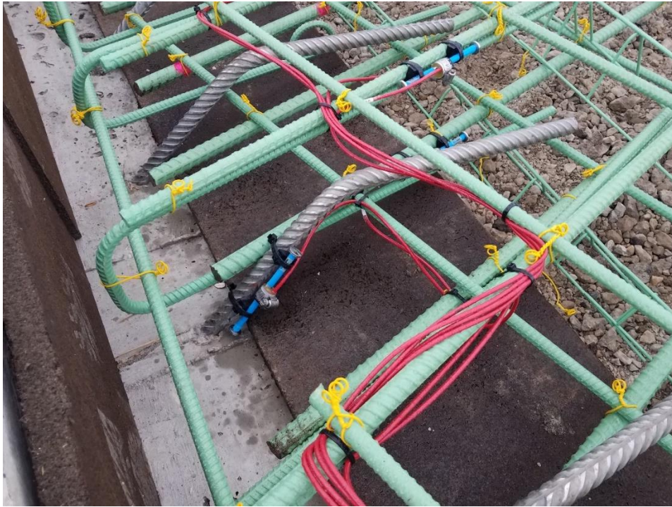
Figure 5.26. Story - Strain Gauges Installed on the Longitudinal Rebar and Tie Bars
