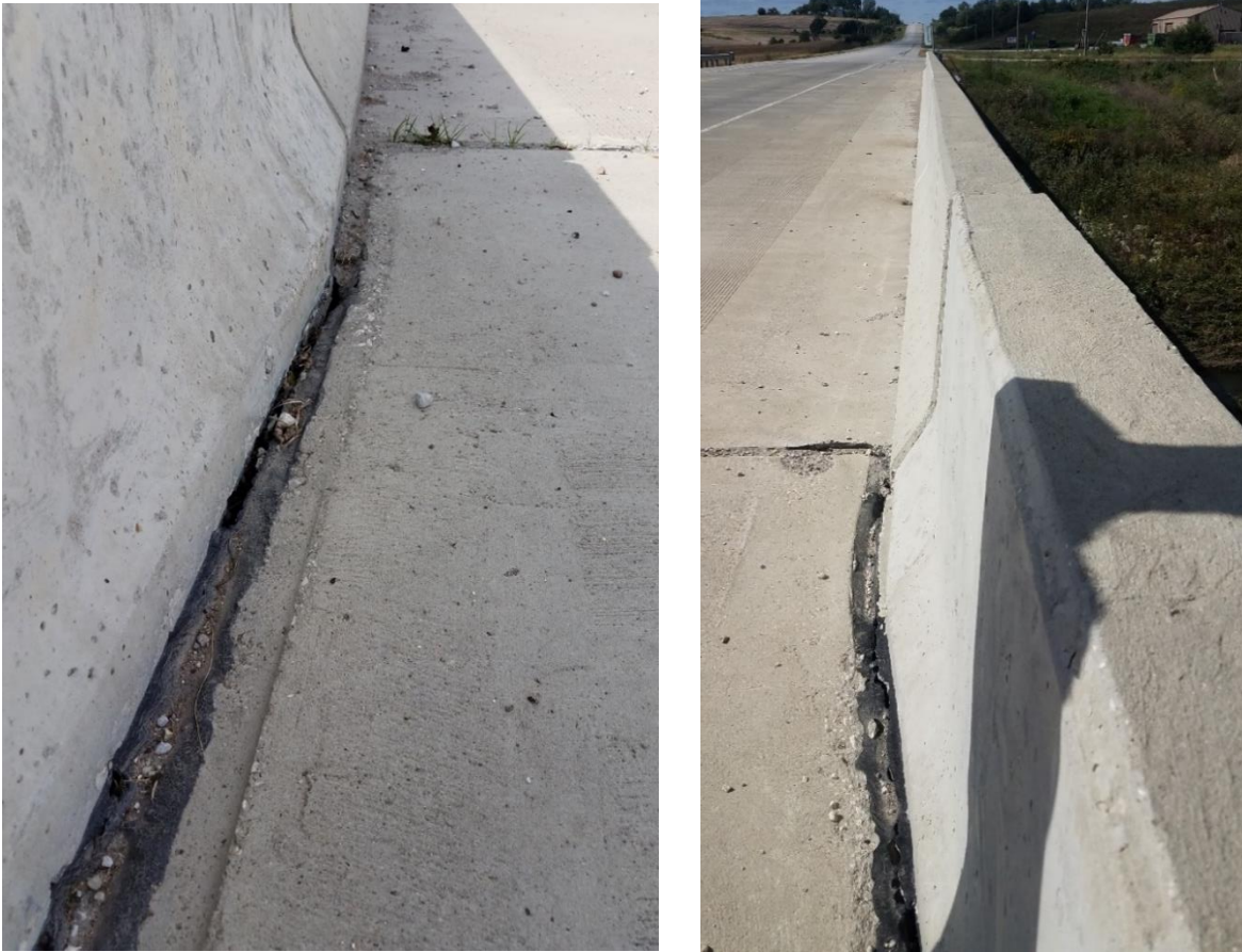
Figure 4.5. (a) Approach Slab to Wingwall Joint Showing Separation (left), (b) Misaligned Wingwall and Barrier (right)
