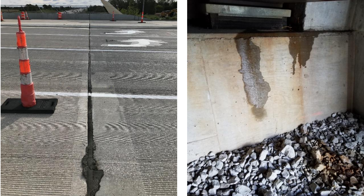
Figure 4.1. (a) South Bridge Deck to Approach Slab Joint with Excess Sealant (left), (b) Water and Abutment Staining at the Outermost Girder (right)
