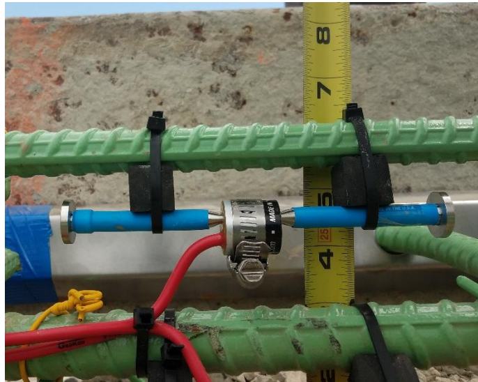
Figure 5.5. Jasper - Typical Strain Gauge Installation
