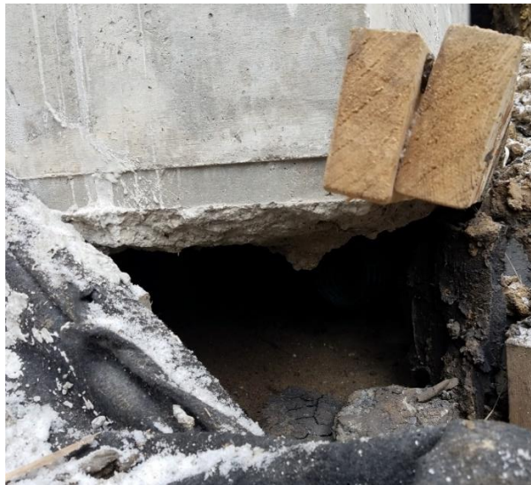
Figure 5.44. Story - Large Void under the South Abutment Corner
