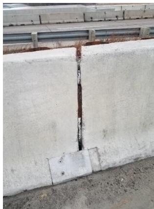
Figure 5.41. Story - Open Barrier Joint (Typical)
