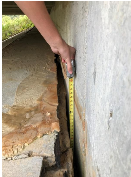
Figure 4.12. Horizontal Void Created by the Embankment Pulling away from the Abutment
