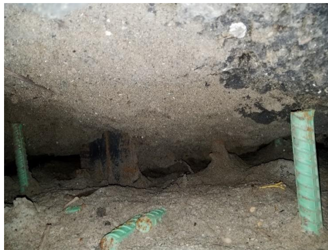
Figure 5.44. Story - Large Void under the South Abutment Corner
