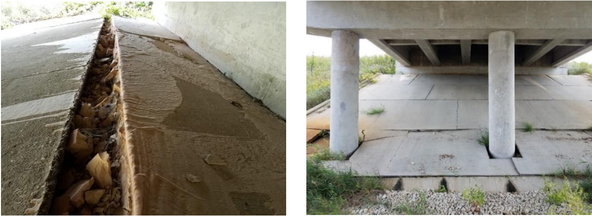
Figure 4.10. (a) Deck to Approach Slab Joint Showing Severe Spalling (left), (b) Additional Deck to Approach Slab Joint Showing Severe Spalling (right)
