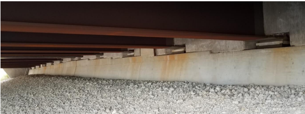
Figure 4.1. (a) South Bridge Deck to Approach Slab Joint with Excess Sealant (left), (b) Water and Abutment Staining at the Outermost Girder (right)
