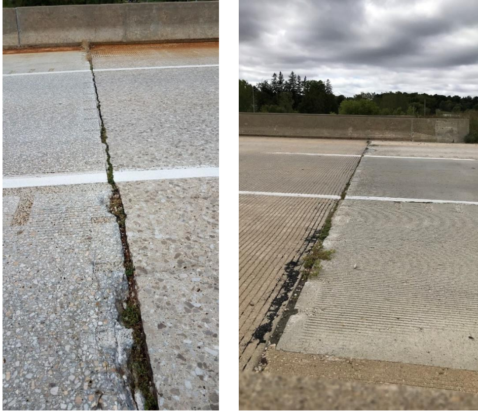
Figure 4.10. (a) Deck to Approach Slab Joint Showing Severe Spalling (left), (b) Additional Deck to Approach Slab Joint Showing Severe Spalling (right)
