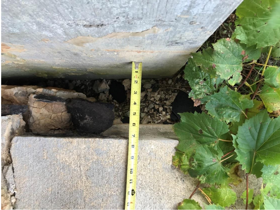
Figure 4.12. Horizontal Void Created by the Embankment Pulling away from the Abutment
